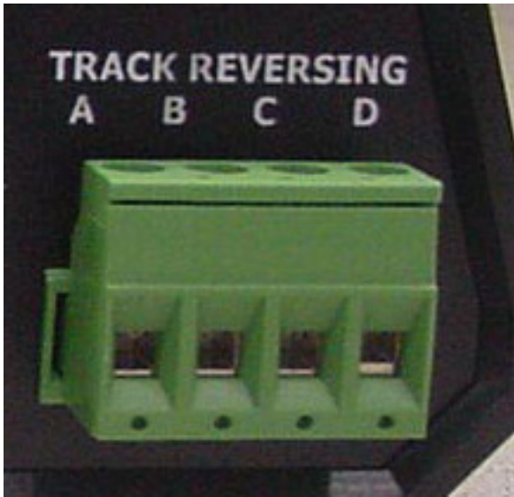
Figure 2: Controller and Bridge Connections
